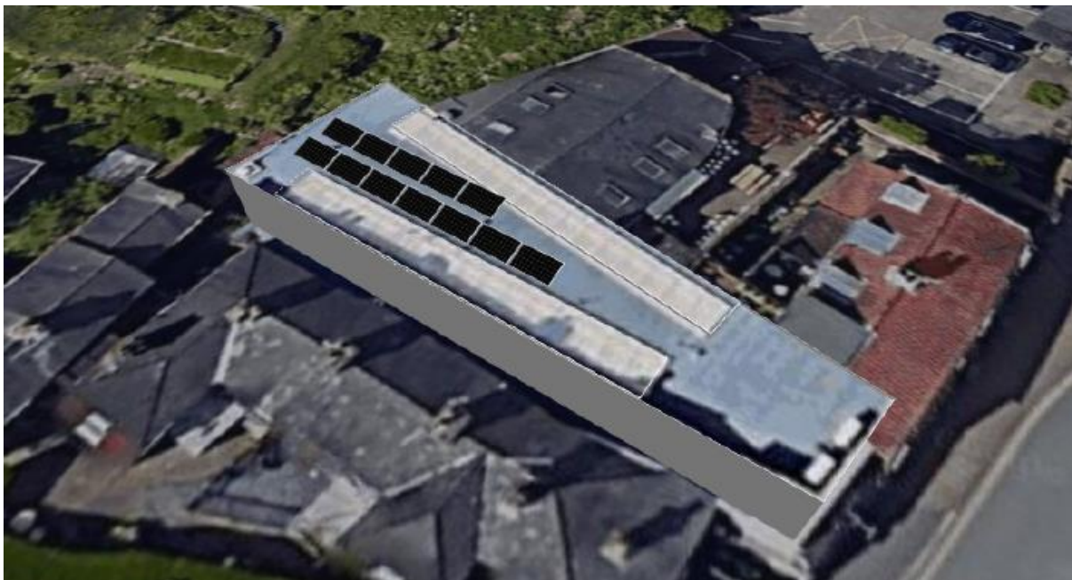
Image to show location of solar panels
